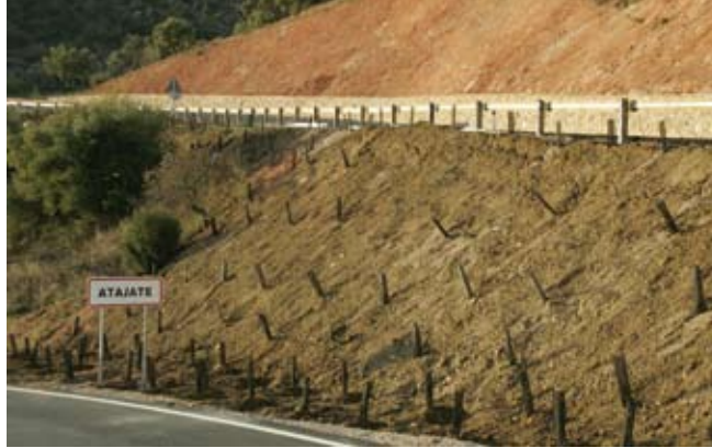
Planting on steep slopes. Revegetation, apart from improving the landscape, is an efficient method of stabilising slopes and protecting them against erosion.
