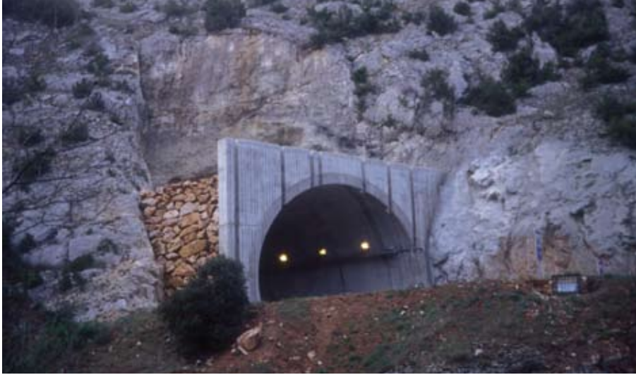
The design of the tunnel portal needs to consider the collapse in the hillside above the final stretch of the tunnel which surrounds the opening. Various strategies are used to camouflage it with ornamental façades or other solutions.
