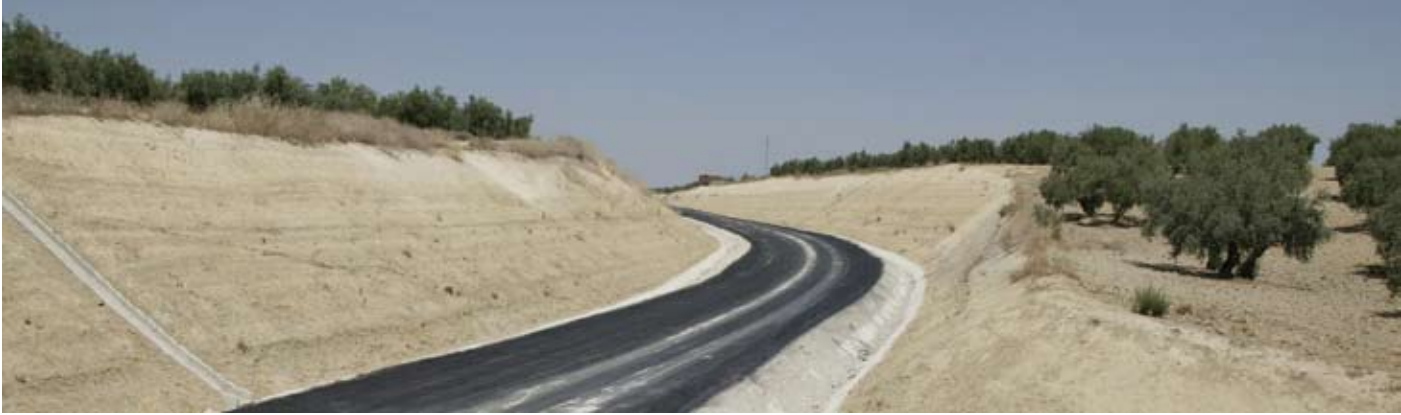
The morphology of excessively geometric embankments with very well defined edges (above) are more imposing than those more irregular and naturalised (below).
