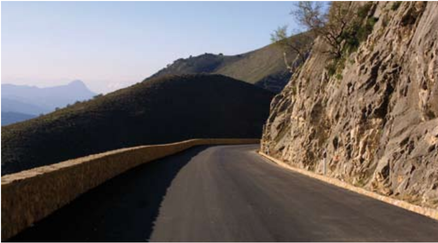
The slope on the right makes revegetation extremely difficult due to its almost vertical layout and lack of soil, although planting can be carried out in excavated hollows.
