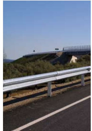
Flexible crash barrier with its characteristic undulating profile and bright metallic geometric design.
