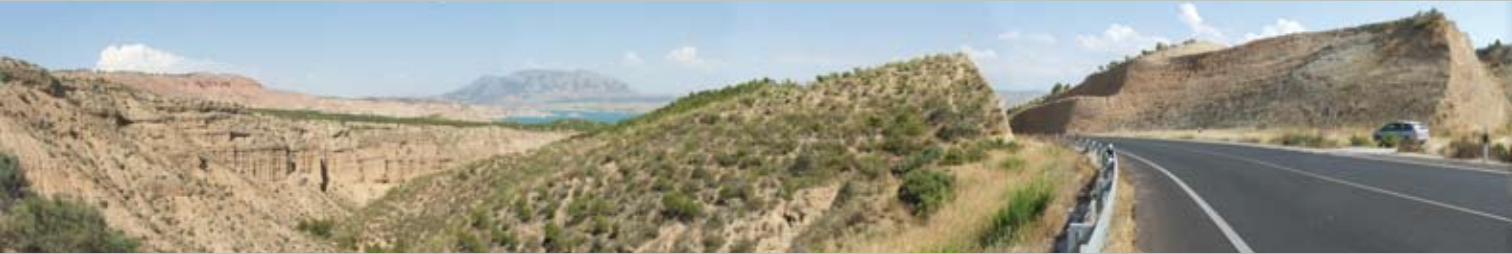
Above, cuttings and berms on the A-315.
