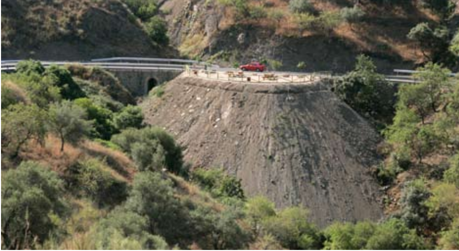
Spoil site next to the road used as a picnic area. The treatment of the sides and the revegetation need to be considered.
