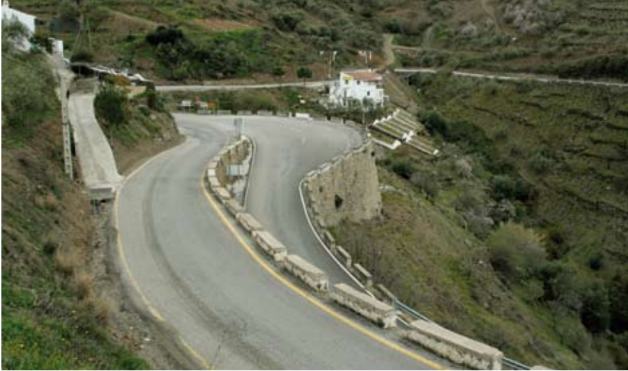
Rigid crash barrier which prevents vehicles from leaving the roadbed. This is a solution for low capacity roads (mountainous, local, or rural roads).
