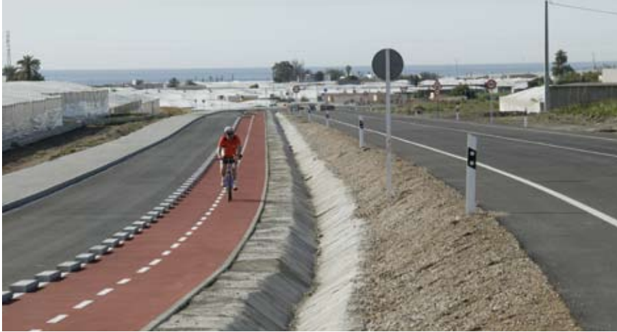
An example of a bicycle lane completely separated from the traffic. The bicycle lane has also been separated and protected from a parallel service road by a discontinuous row of kerbstones, whilst pedestrians are served by a footpath (far left of the picture).
