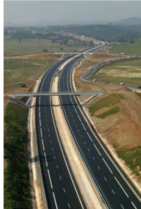
The A-381 Jerez-Los Barrios (Cádiz). The geometric parameters of the layout (gradient, curve radius, stopping sight distance) determine driving safety and comfort as well as its presence (linearity, sinuousness) in the landscape.
