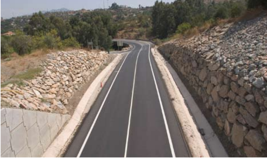
The retaining walls made from precast pieces (bottom left-hand corner of the picture) clash with more natural finishes, such as the rockfill wall on the right and the excavation on the left.
