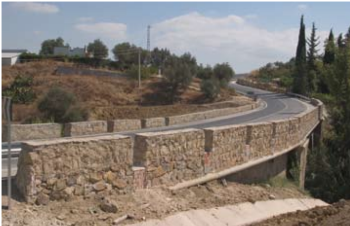
The flexible crash barrier has been replaced on this bridge by a rigid crenellated parapet.
