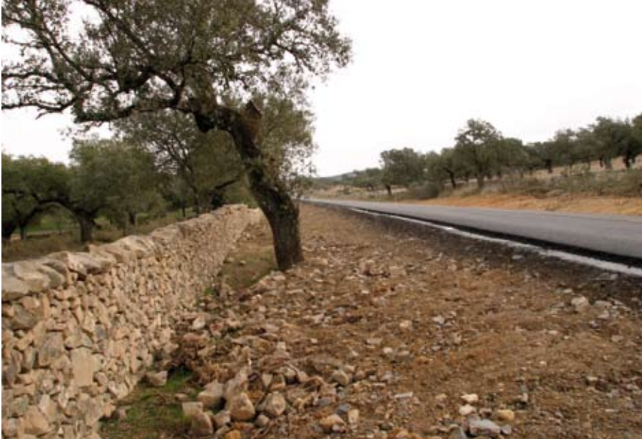
A dry stone wall marks the edge of an estate. Imitating these character references when installing retaining elements can give identity to the road infrastructure.
