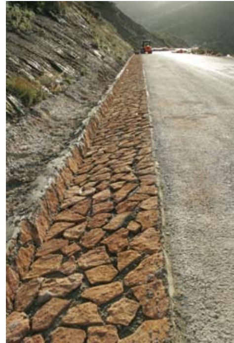
Riprap drainage ditch. This is an alternative which integrates better with the surroundings than concrete lined or precast elements.
