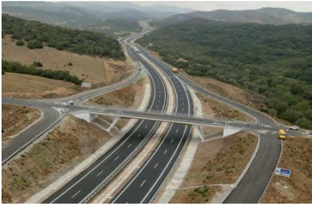
Junctions have to be studied in detail, analysing the position of slip roads and roundabouts relative to the main roadway and the setting, avoiding heavy alterations to the surroundings and preserving views.
