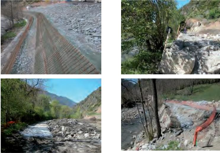
Figure 22: Top left-hand photograph: reinforced earth wall; other photographs: stone wall.
